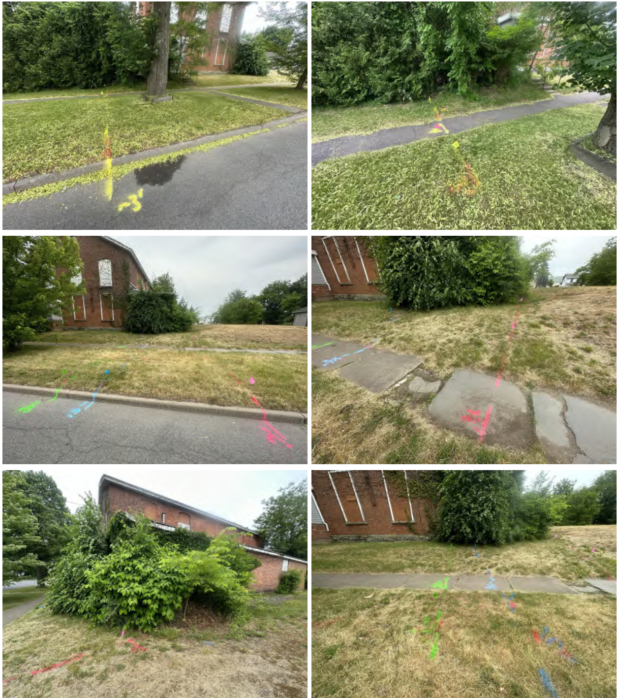
Fig. 5: Images of the gas, water, and sewer for the main building; as well as the unconfirmed utility/unknown linear anomaly that was detected at the southeast side of the property - near the water and sewer.
