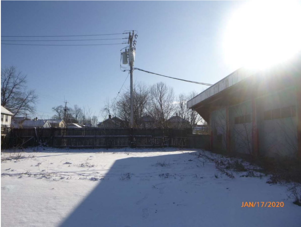
Photo 49. View of the back (north side) of the building.
