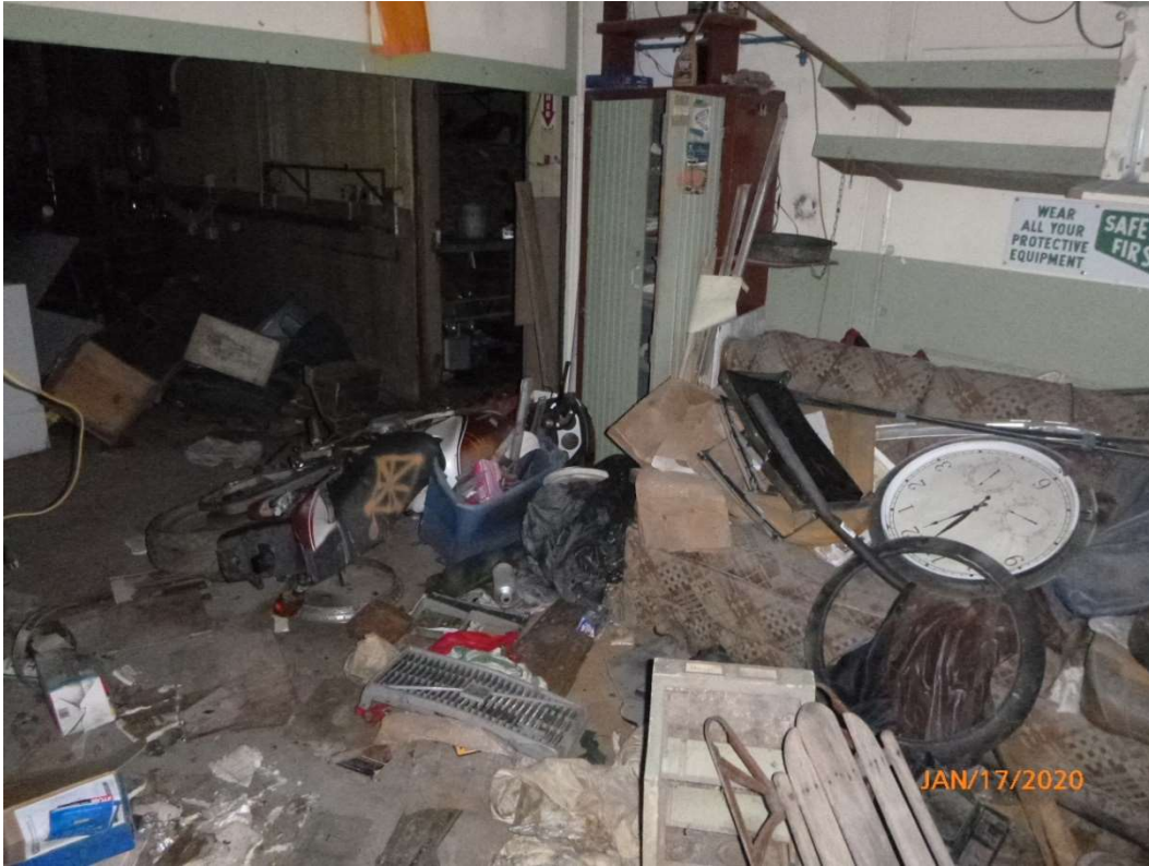
Photo 39. View looking at the west wall of the shop.
