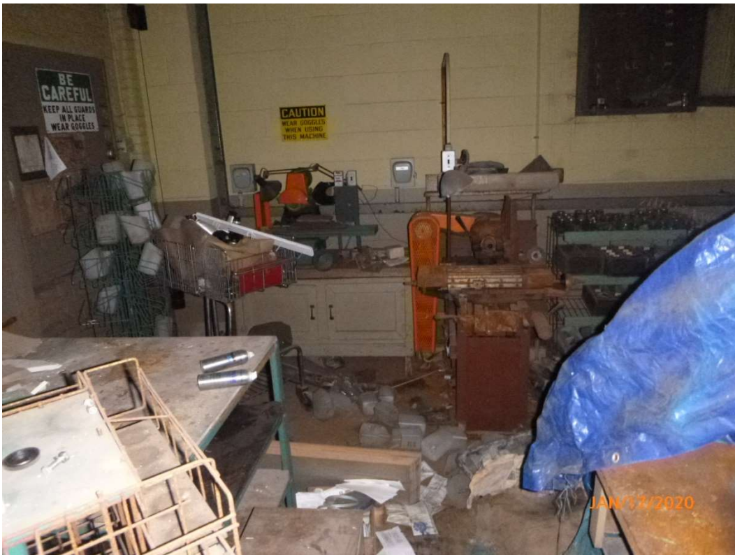
Photo 38. View of the south west corner of the shop area of the building.
