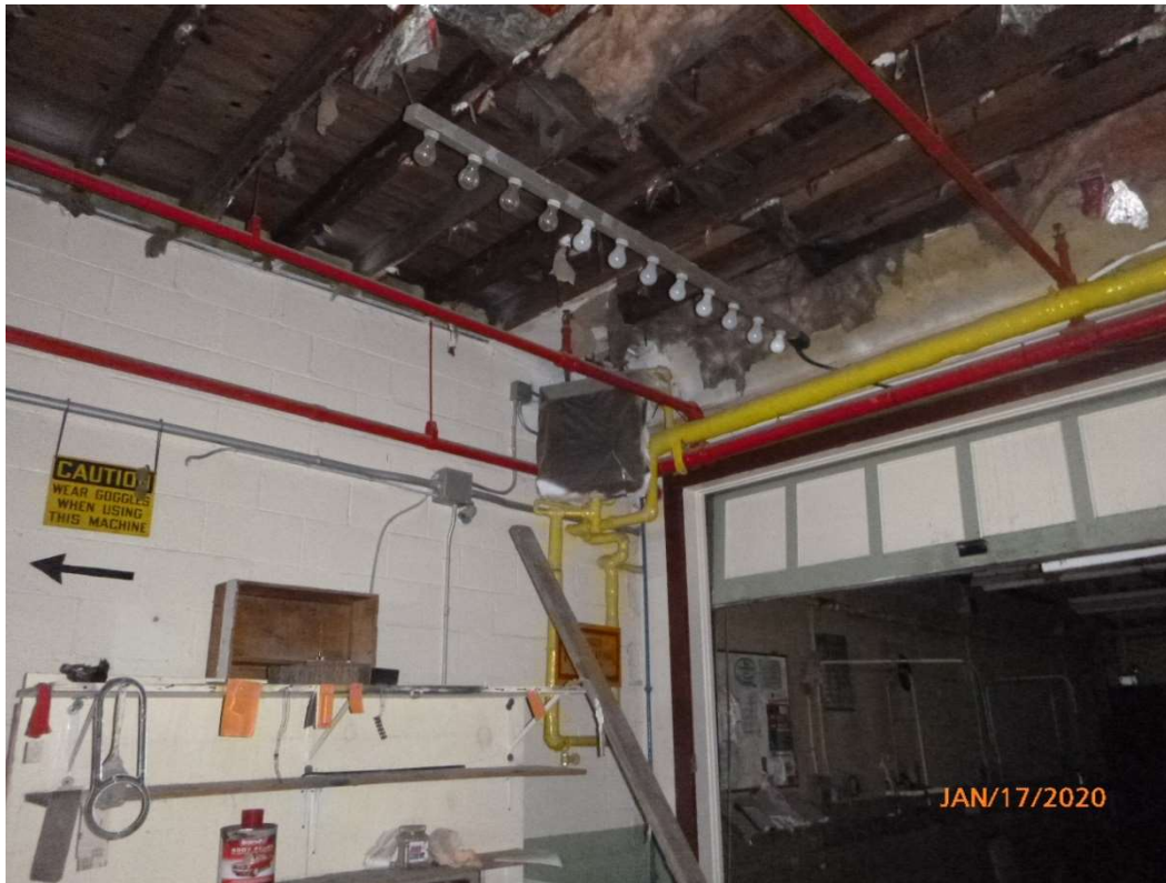
Photo 43. Heater in the southeast corner of the shop.
