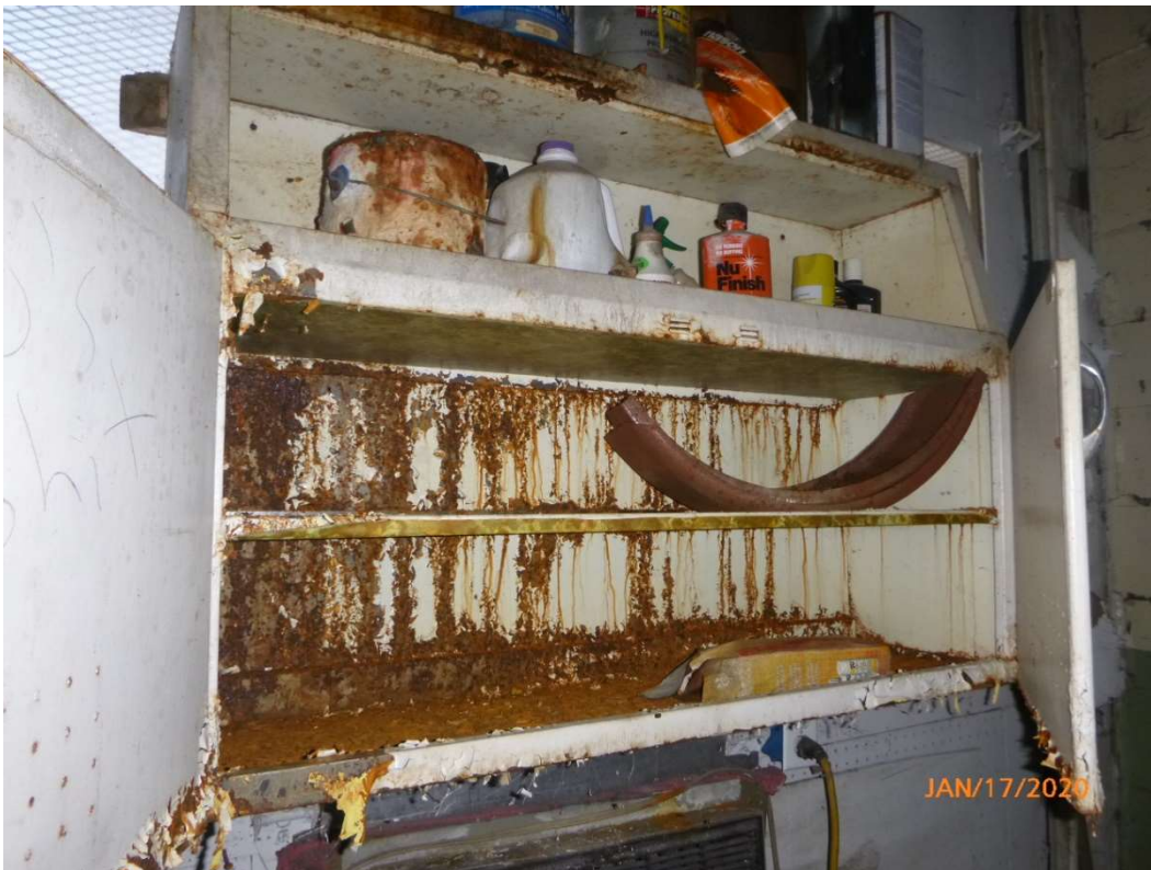
Photo 42. Presumed storage of solvents/chemicals in the shop along the north wall of the building.
