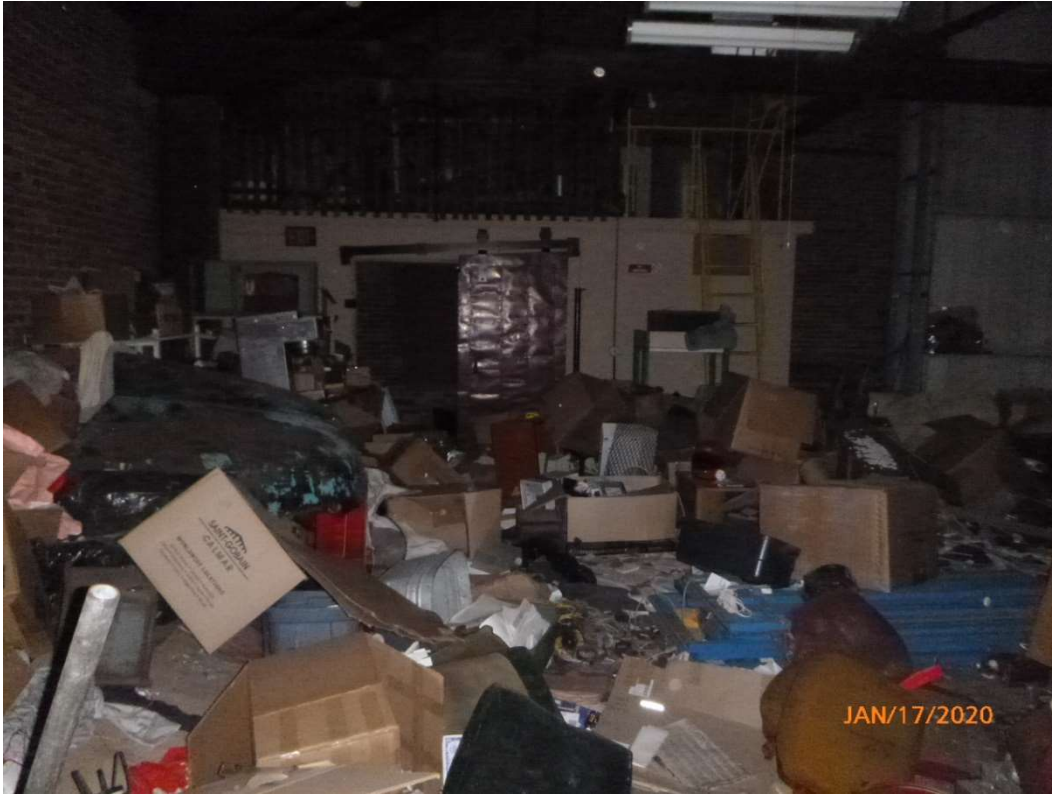
Photo 1. Second floor storage area on the second floor looking toward the front of the building.
