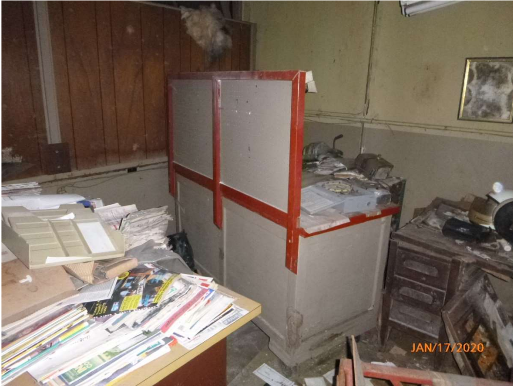
Photo 15. Cubicle office space along the east wall of the building.
