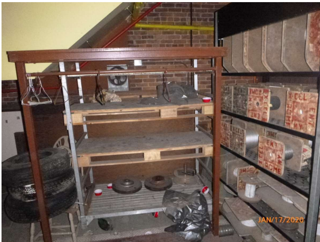
Photo 22. More storage and spools in the manufacturing room along the west wall of the building.
