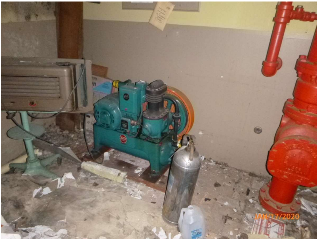
Photo 12. York heat pump located in the sprinkler system room.
