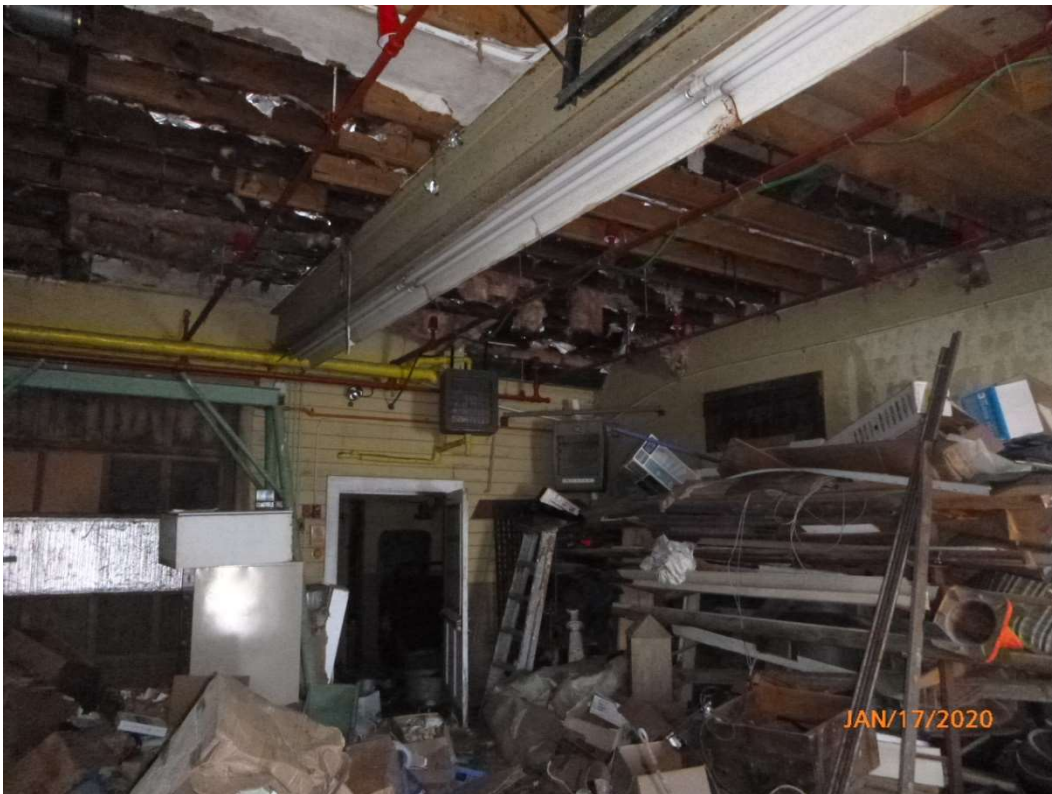
Photo 46. Heater in the northwest corner room of the building.
