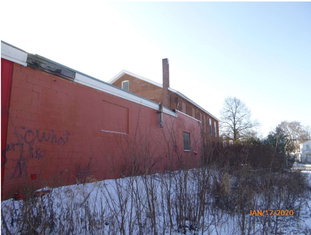
Photo 50. View of the west side of the building.
