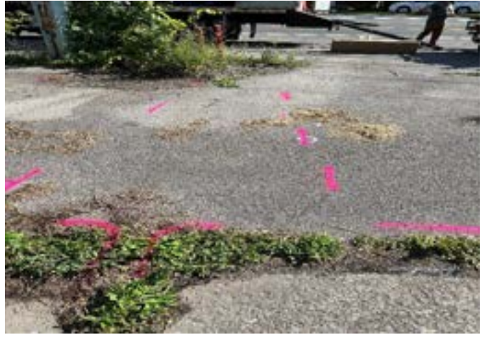
View of UST lines to canopy identified during GPR activities facing north.
