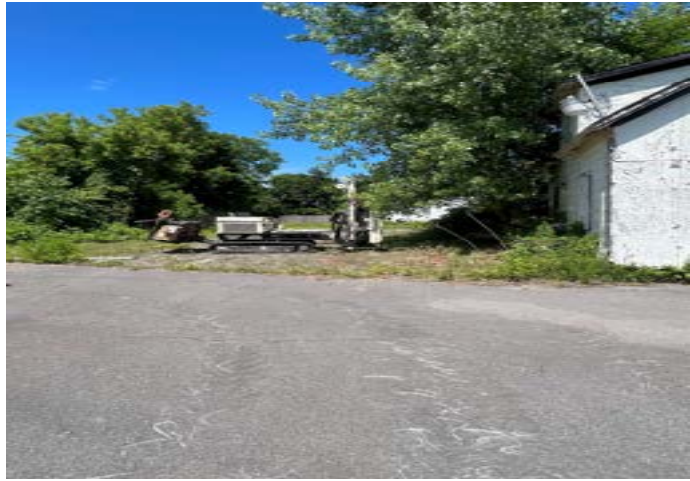
View of geoprobe activities facing west.
