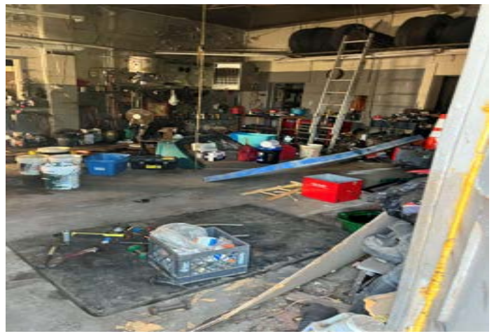
View of inside the Commercial building garage.
