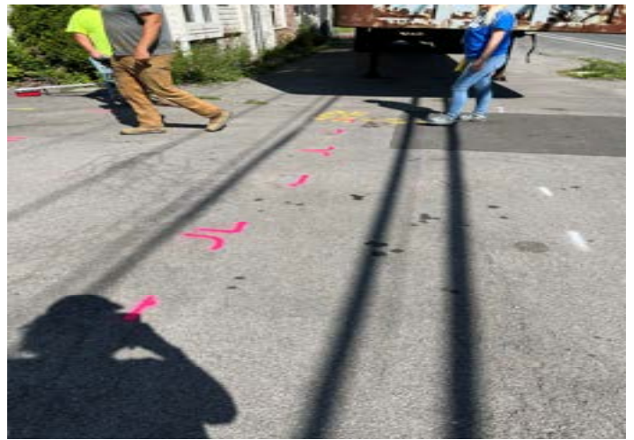
View of four USTs, gas and sewer lines identified during GPR activities facing west.
