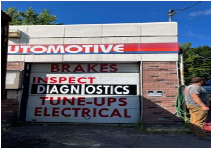
View of garage door of the Commercial building facing south.
