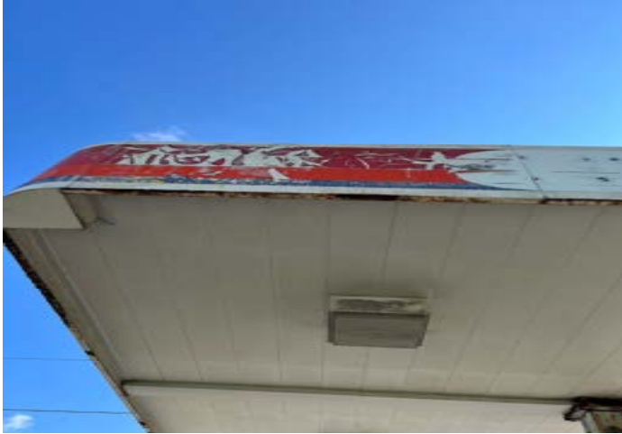
View of existing dispenser canopy located east of the Commercial building.
