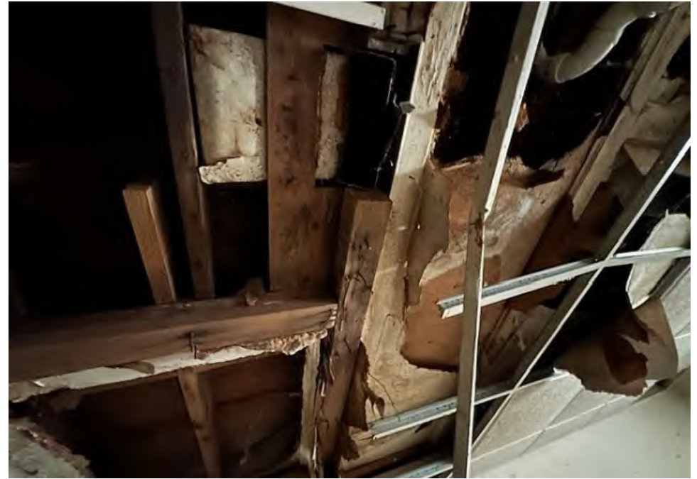
room #1 - duct wrap
