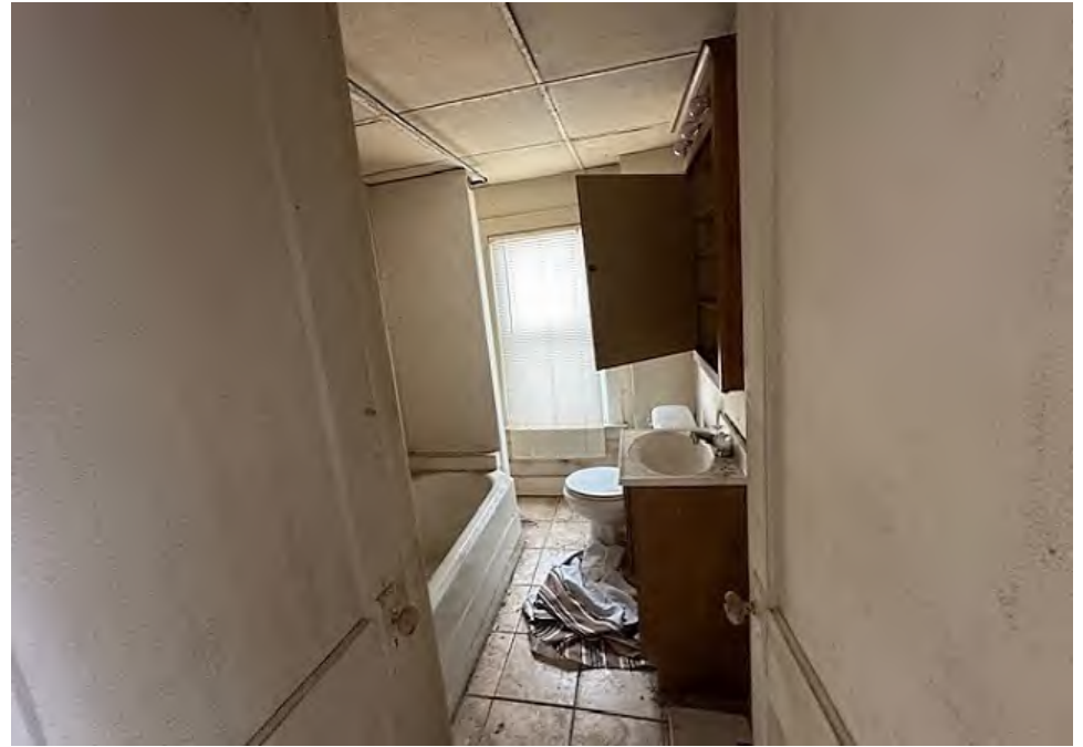
2nd floor - bathroom
