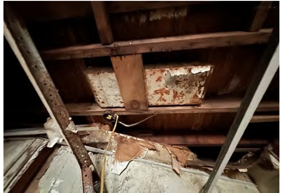
room #1 - duct wrap
