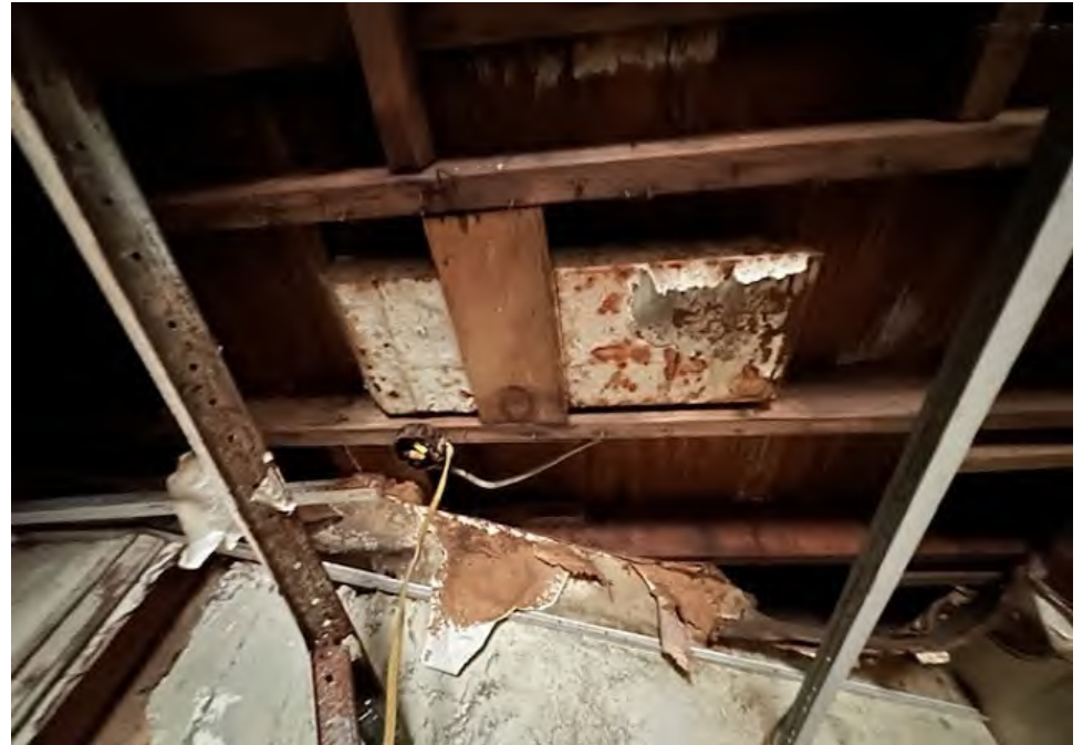
room #1 - duct wrap
