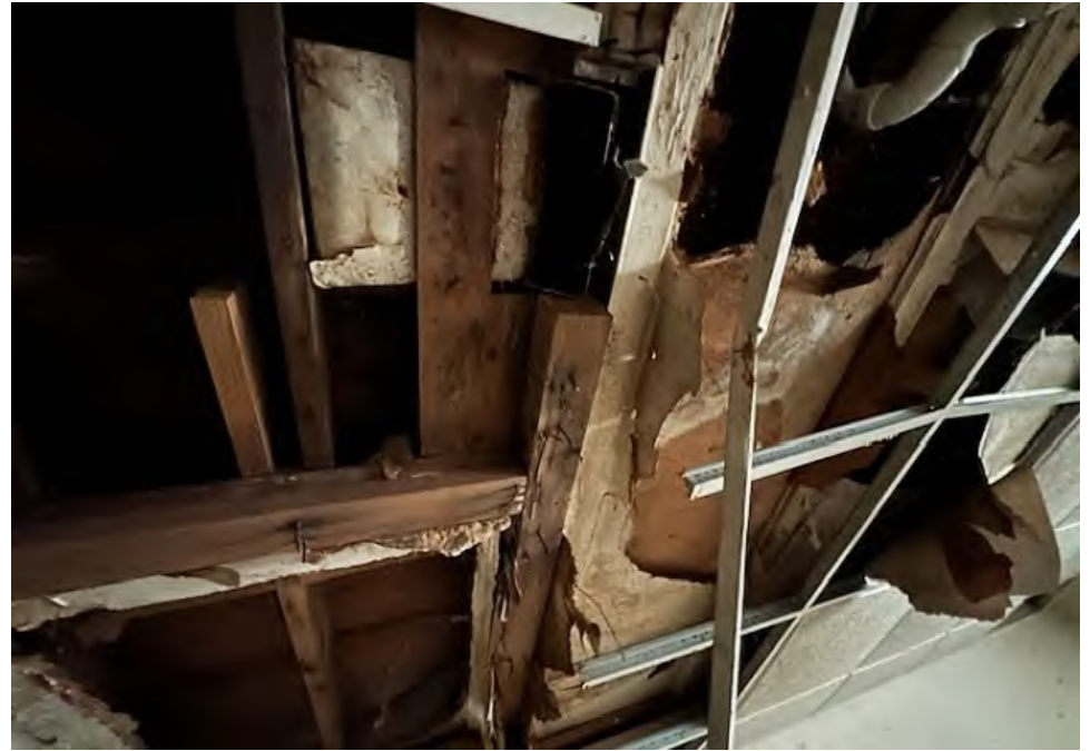
room #1 - duct wrap
