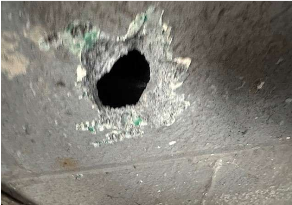
Garage wall - no vermiculite
