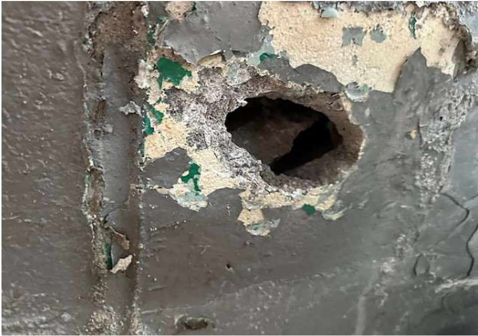
Garage wall - no vermiculite
