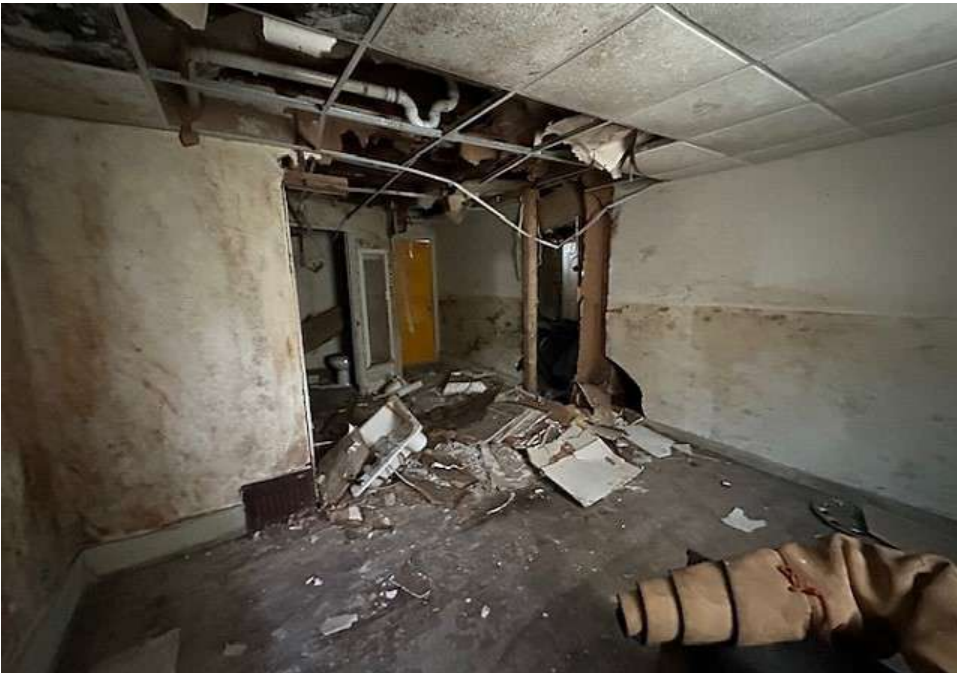
room #1 - debris pile
