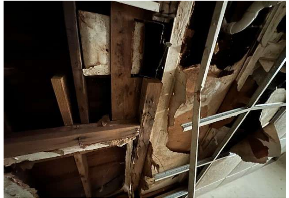
room #1 - duct wrap
