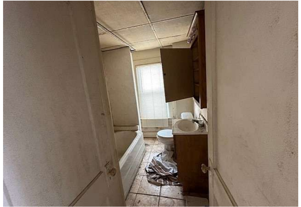
2nd floor - bathroom
