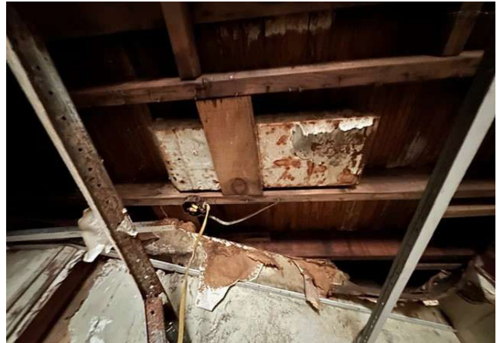
room #1 - duct wrap
