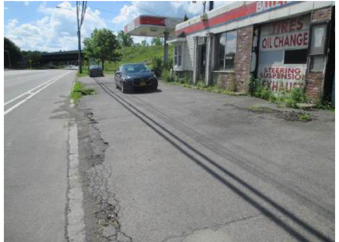
View of Commercial building from the front facing east.
