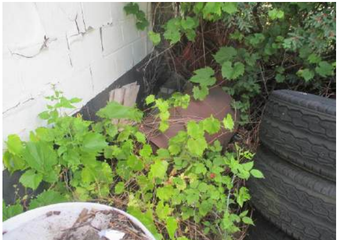
View of 55-gal steel drum and tires behind servicing garage.
