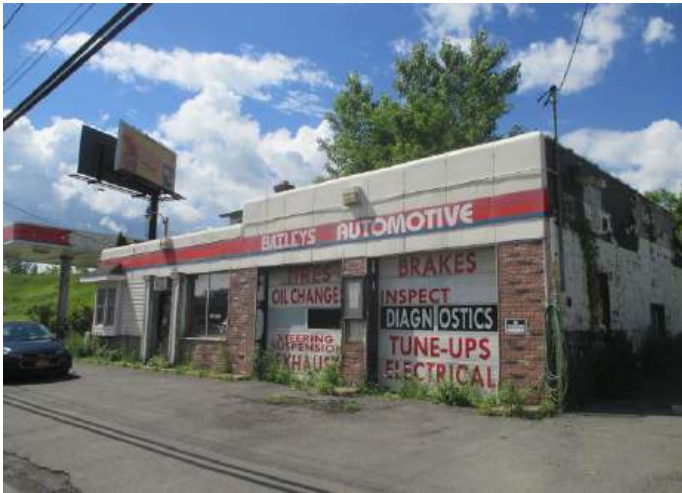
View of Commercial building from the front facing southeast.
