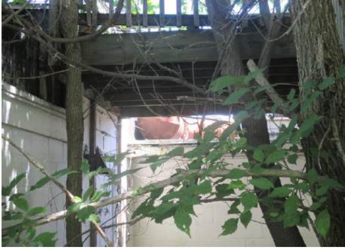
View of roof of Commercial building with two 55-gal drums.
