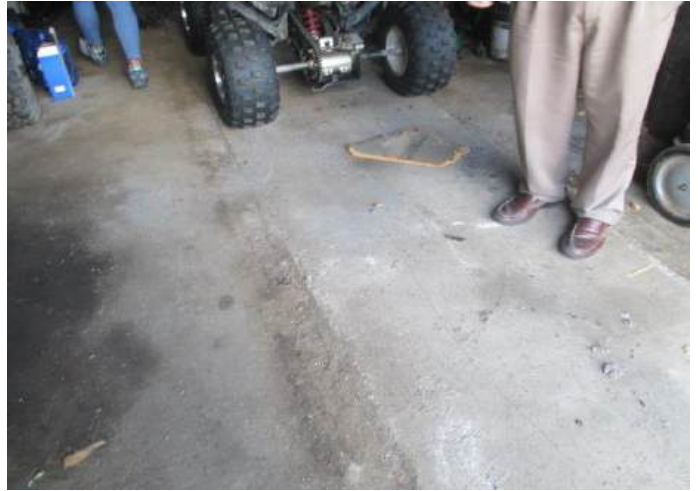
View of inside garage area of Commercial building concrete patched area.
