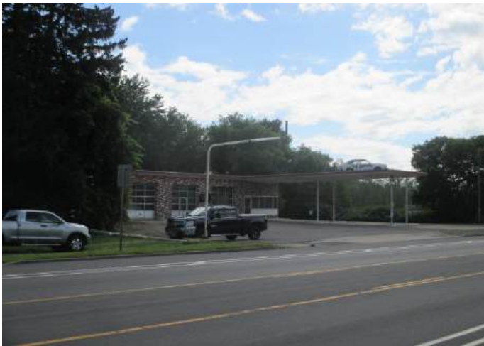
View of adjacent property facing northeast.
