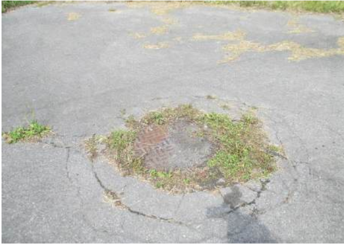
View of municipal sewer manhole on-site.
