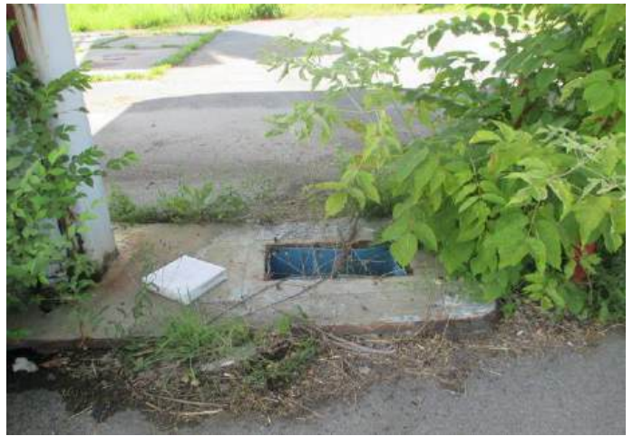
View of former gasoline dispenser located beneath canopy on the northeastern side of Site.
