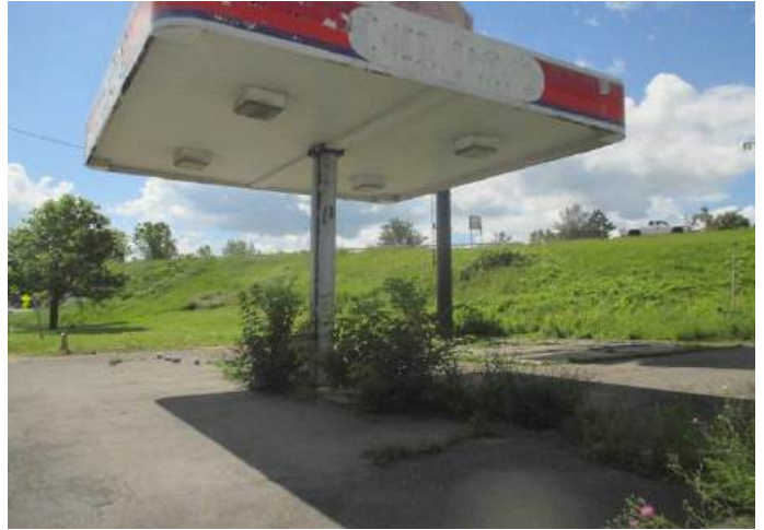
View of fill station canopy.
