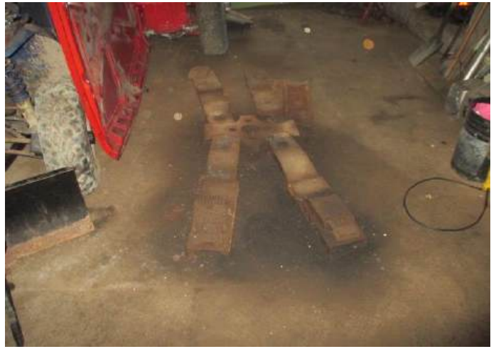
View of inside garage area of Commercial building floor lift.
