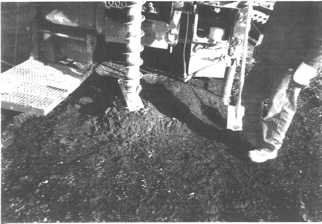
Characterizing Materials in the Wood Chip Pile – Location No. 2
