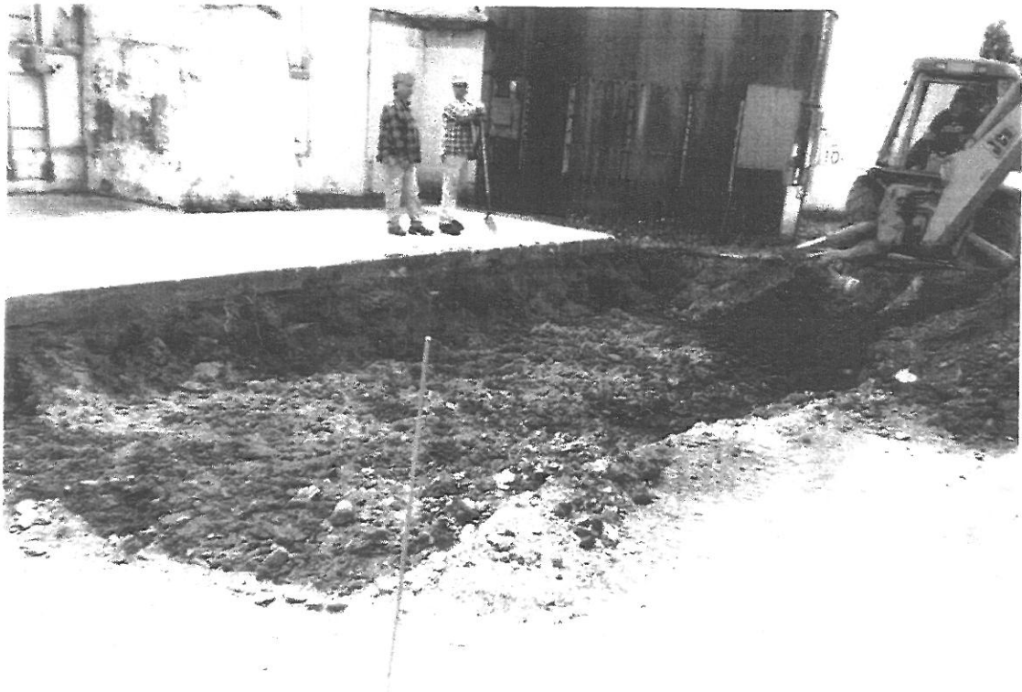
Former UST Area Excavation Adjacent to Boiler House No. 5
