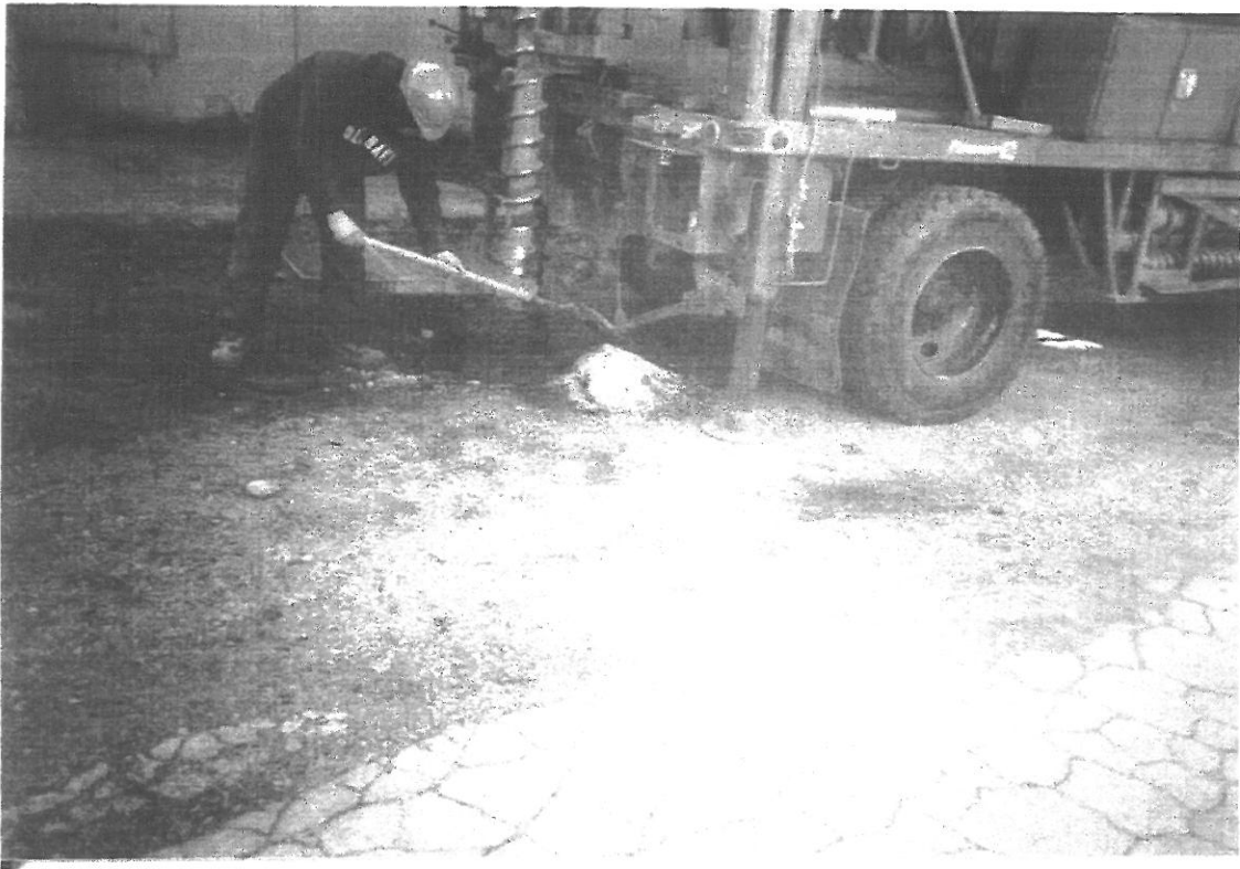
Former UST Area Adjacent to Boiler House No. 5
