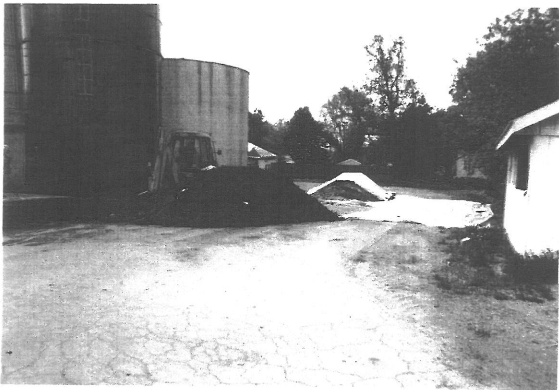
Former UST Area Excavation Adjacent to Boiler House No. 5
